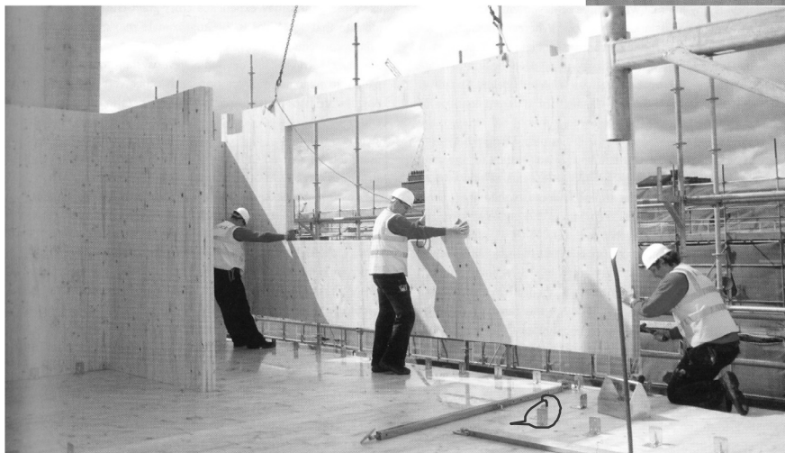
“Honeycomb” construction in UK
