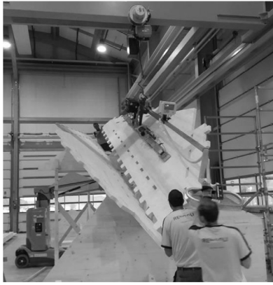
Shell assembly at fabrication shop
