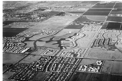
EXPOSURE C OPEN TERRAIN WITH SCATTERED OBSTRUCTIONS HAVING HEIGHTS GENERALLY LESS THAN 30 FT FOR MOST WIND DIRECTIONS. ALL 1-STORY STRUCTURES WITH A MEAN ROOF HEIGHT LESS THAN 30 FT IN THE PHOTOGRAPH ARE LESS THAN 1500 FT OR TEN TIMES THE HEIGHT OF THE STRUCTURE, WHICHEVER IS GREATER, FROM AN OPEN FIELD THAT PREVENTS THE USE OF EXPOSURE B
