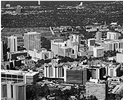
EXPOSURE B STRUCTURES IN THE FOREGROUND ARE LOCATED IN EXPOSURE B. STRUCTURES IN THE CENTER TOP OF THE PHOTOGRAPH ADJACENT TO THE CLEARING TO THE LEFT, WHICH IS GREATER THAN 200 M IN LENGTH, ARE LOCATED IN EXPOSURE C WHEN WIND COMES FROM THE LEFT OVER THE CLEARING (SEE FIGURE C6-5)
