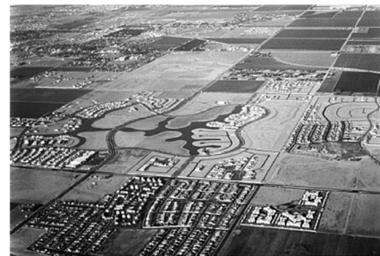
EXPOSURE C FLAT TERRAIN WITH SCATTERED OBSTRUCTIONS HAVING HEIGHTS GENERALLY LESS THAN 30 FT FOR MOST WIND DIRECTIONS. ALL 1-STORY STRUCTURES WITH A MEAN ROOF HEIGHT LESS THAN 30 FT IN THE PHOTOGRAPH ARE LESS THAN 1500 FT OR TEN TIMES THE HEIGHT OF THE STRUCTURE, WHICHEVER IS GREATER, FROM AN OPEN FIELD THAT PREVENTS THE USE OF EXPOSURE B
