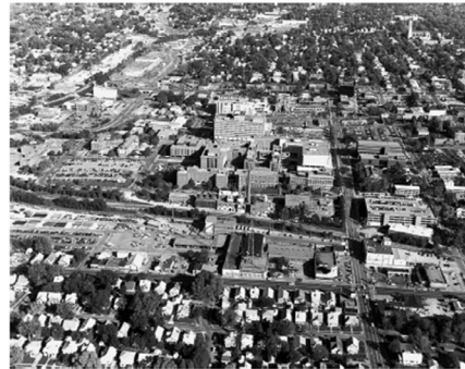
EXPOSURE B URBAN AREA WITH NUMEROUS CLOSELY SPACED OBSTRUCTIONS HAVING THE SIZE OF SINGLE-FAMILY DWELLINGS OR LARGER. FOR ALL STRUCTURES SHOWN, TERRAIN REPRESENTATIVE OF SURFACE ROUGHNESS CATEGORY B EXTENDS MORE THAN TEN TIMES THE HEIGHT OF THE STRUCTURE OR 800 M, WHICHEVER IS GREATER, IN THE UPWIND DIRECTION
