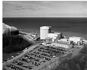
EXPOSURE D A BUILDING AT THE SHORELINE (EXCLUDING SHORELINES IN HURRICANE-PRONE REGIONS) WITH WIND FLOWING OVER OPEN WATER FOR A DISTANCE OF AT LEAST 1 MILE. SHORELINES IN EXPOSURE D INCLUDE INLAND WATERWAYS, THE GREAT LAKES, AND COASTAL AREAS OF CALIFORNIA, OREGON, WASHINGTON, AND ALASKA
