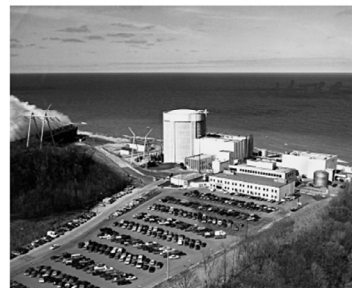
EXPOSURE D A BUILDING AT THE SHORELINE (EXCLUDING SHORELINES IN HURRICANE-PRONE REGIONS) WITH WIND FLOWING OVER OPEN WATER FOR A DISTANCE OF AT LEAST 1 MILE. SHORELINES IN EXPOSURE D INCLUDE INLAND WATERWAYS, THE GREAT LAKES, AND COASTAL AREAS OF CALIFORNIA, OREGON, WASHINGTON, AND ALASKA
