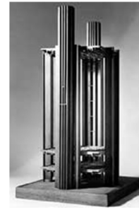
Louis I. Kahn's structural model for the Richards Medical Research Laboratory
