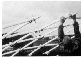
6.16 Assembly of the grid elements
